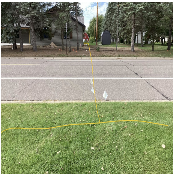
Gas service route flagged
